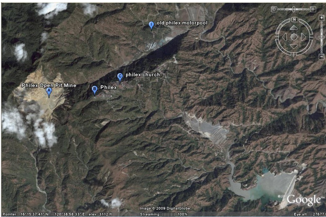
Figure 42. Philex open pit mine, tailing ponds, and nearby areas on Google Earth (labels are from Google Earth and not by the author of this work)
