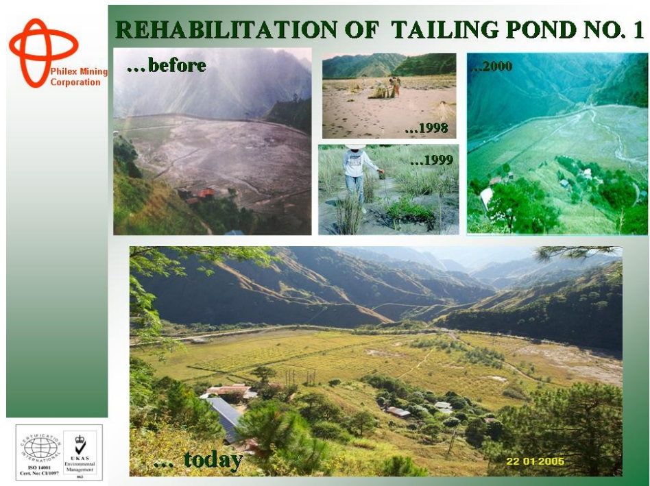
Figure 46. Philex tailings pond 1 then and now (26 hectares, expected useful life was 10 years, closed in 1981)
